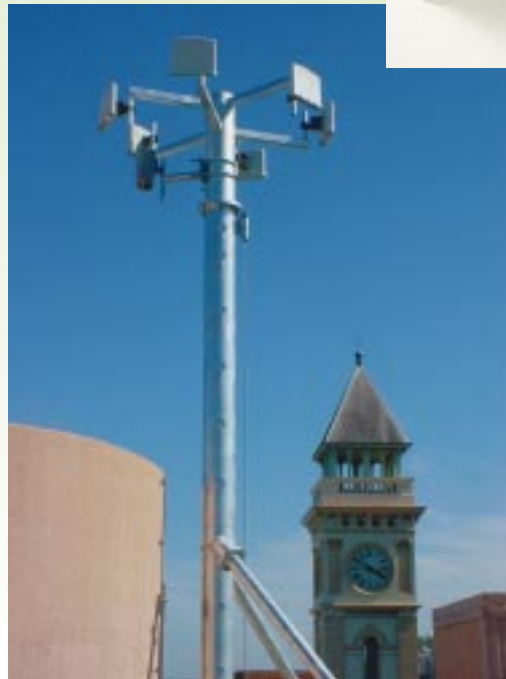
Six-sectored WipLL base station configuration
